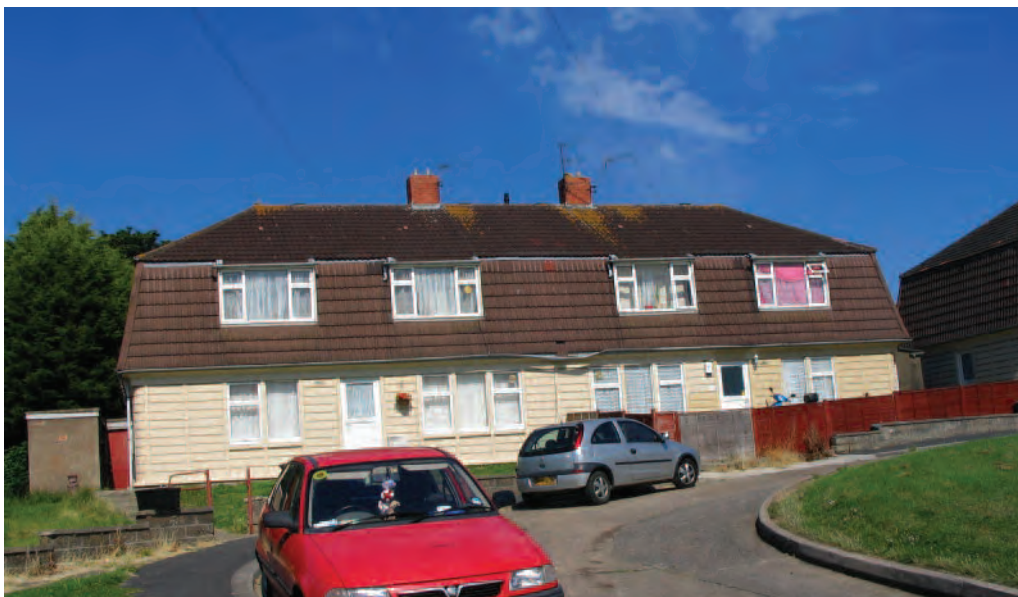
A pair of maisonettes in a 'Cornish House' In Lockleaze
