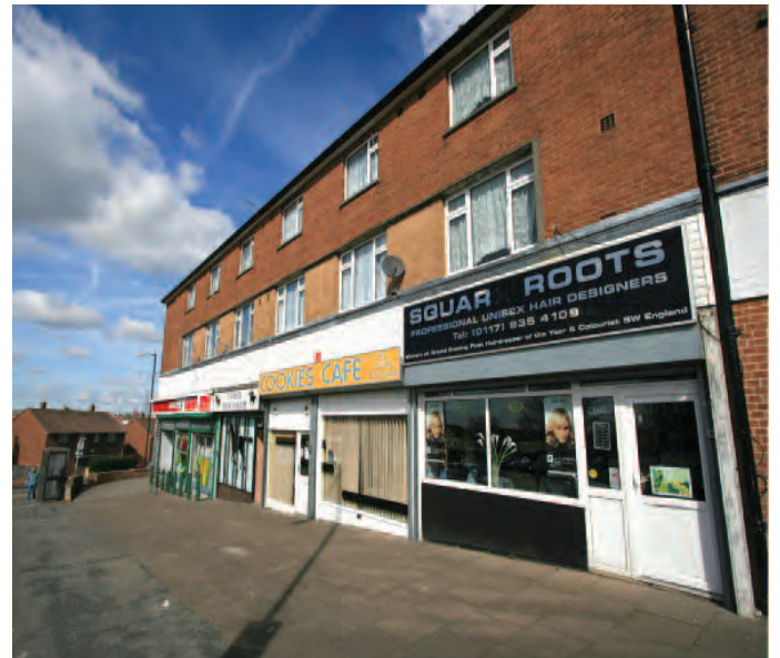
Retail at Gainsborough Square
